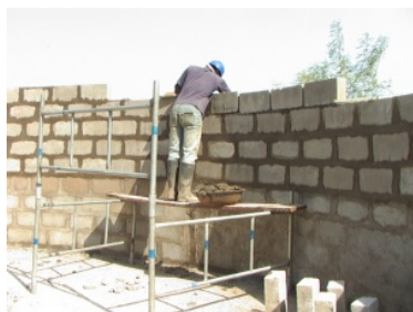
Block Wall Construction
